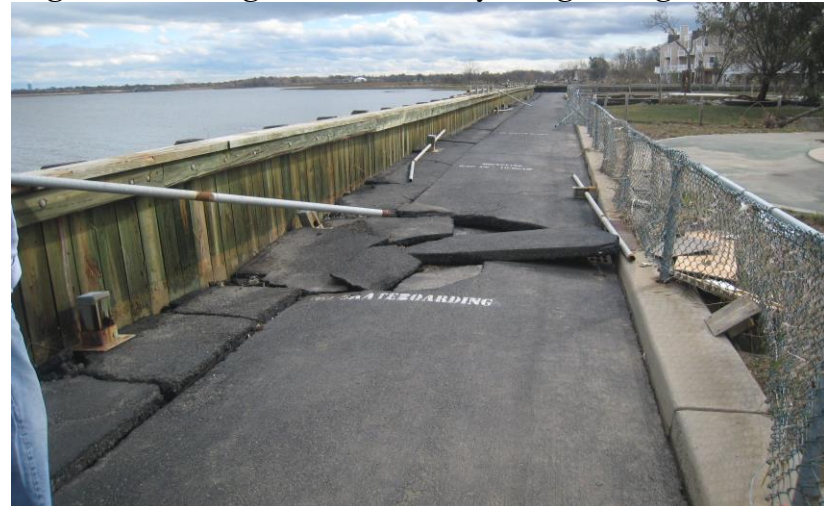
Figure 14: Damage to the Walkway along Firefighter's Park
