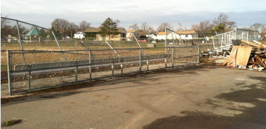
Figure 13: Damages and Debris at Scholer Park
