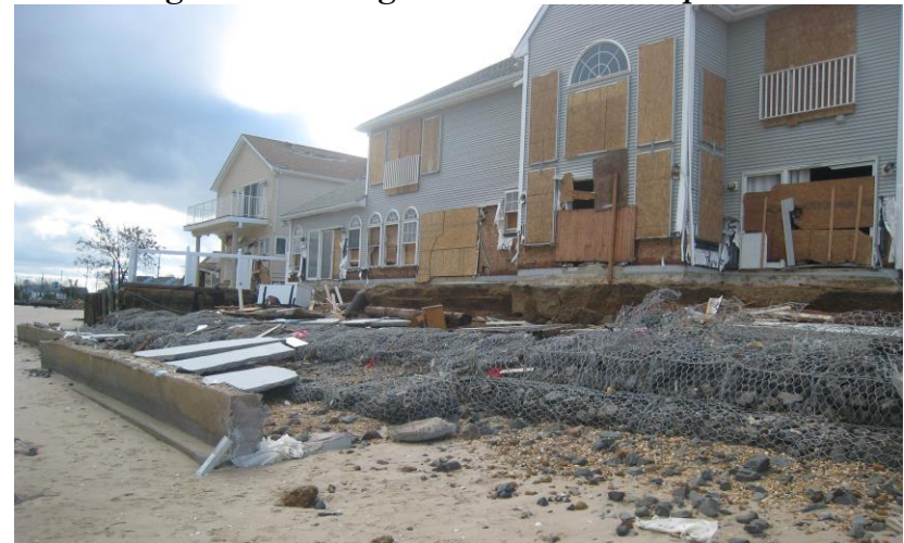
Figure 17: Damage to Beachfront Properties
